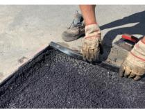
Corabit Joint tape is a fusible bitumenbased joint tape developed for road construction.
